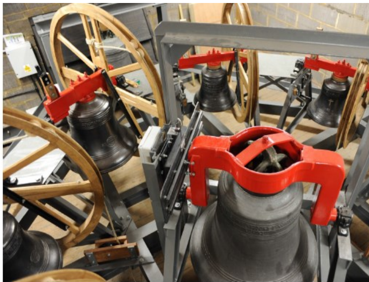
NEW PEAL OF EIGHT IN RADIAL FRAME TOGETHER WITH ELECTRICALLY SWUNG BOURDON AND STATIONARY SERVICE BELL, SOUTH OCKENDON.
